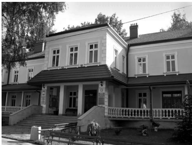
Fig. 6. Building housing the State School of Higher Vocational Education President's Office (photo: J. Kobylarczyk)
