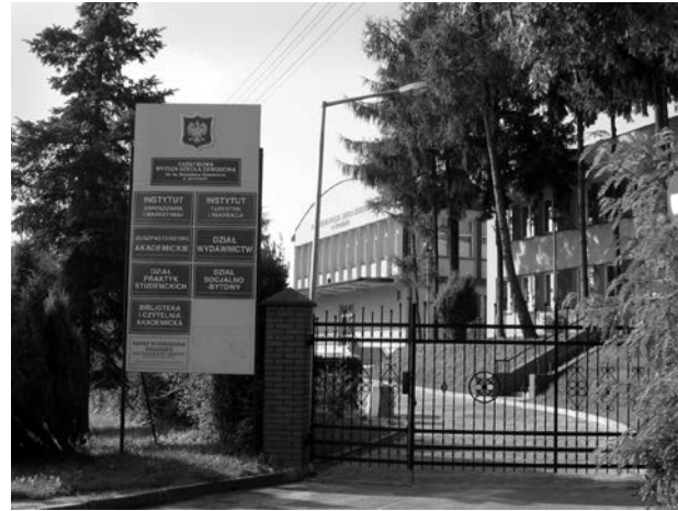
Fig. 7. Main entrance to the State School of Higher Vocational Education (photo: J. Kobylarczyk)
