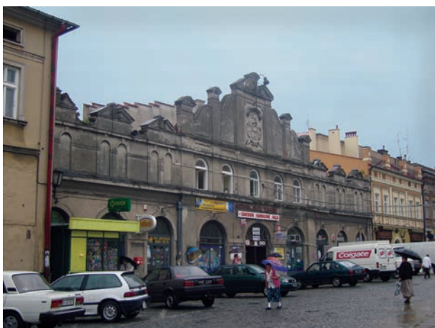
Fig. 2. Market hall – roofed courtyard (photo: J. Kobylarczyk)
