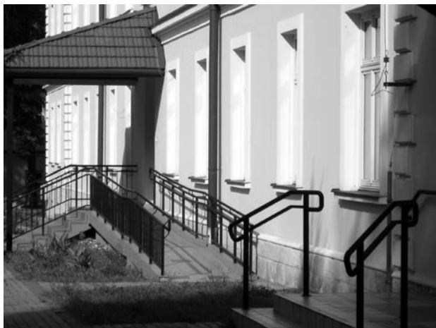
Fig. 9. Adjustment of the school for the needs of the disabled persons (photo: J. Kobylarczyk)
