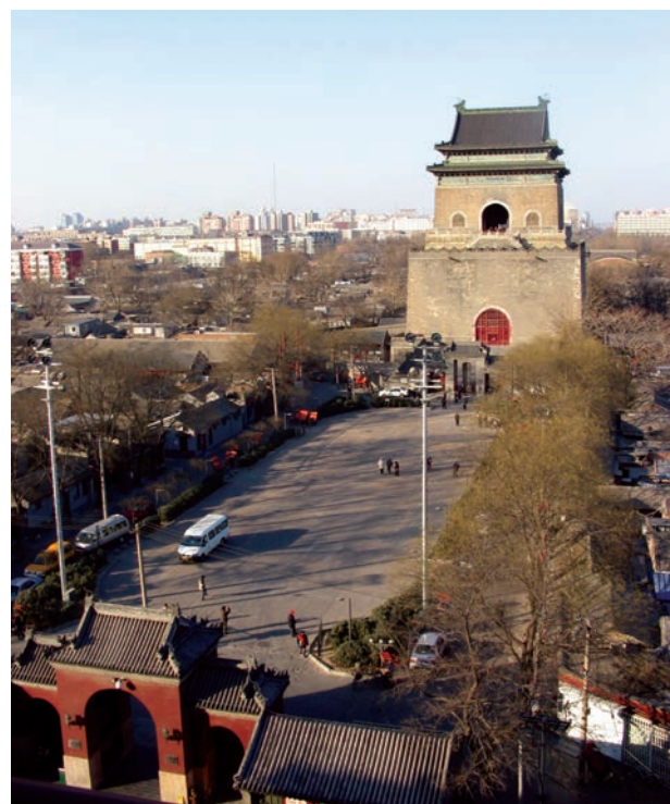
Fig. 7. The Bell Tower with the square preceding it from the south (photo: J. Krajewska)
