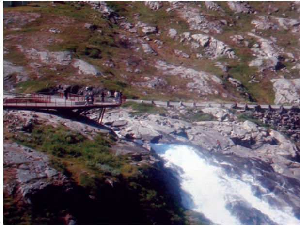
Fig. 1. Trollstigplatået Geiranger – Trollstigen (arch. Reiulf Ramstad Arkitekter AS, under realization 2004–2010) – light steel construction finished with wood enabling observation of Troll Road (photo: E. Cisek)
