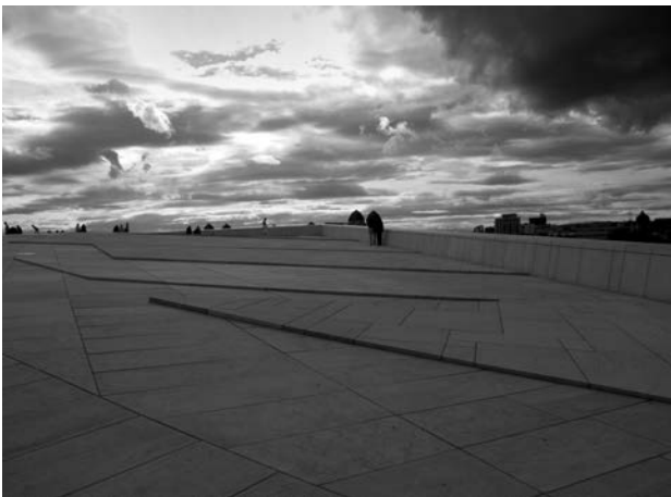
Fig. 9. Den Norske Opera & Ballet in Bjørvika in Oslo (arch. Snøhetta, realization in 2008) – the roof of the Opera House covered with marble slabs (photo: E. Cisek)
