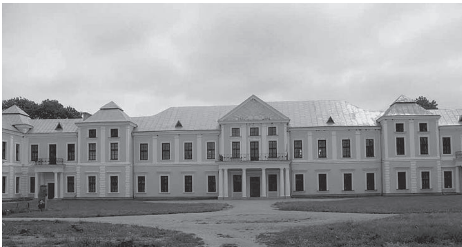
Fig. 4. Palace in Vyshnivets. Overall view from the courtyard
