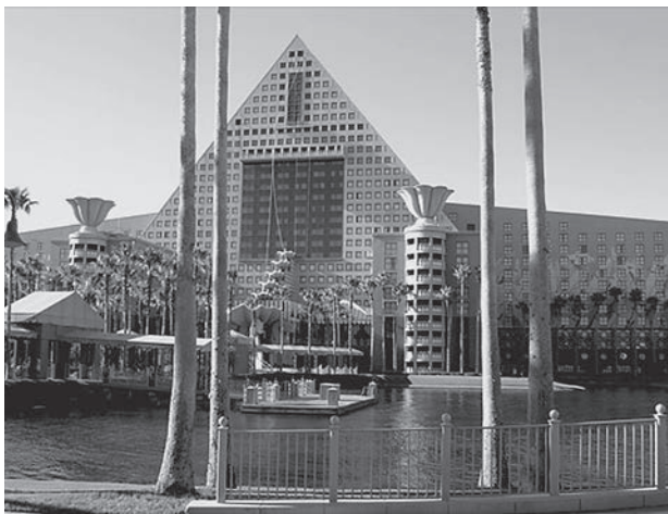
Fig. 1. Dolphin and Swan Hotels in Walt Disney World, Orlando 1990. Architect Michaela Graves
