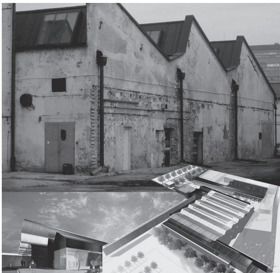
Fig. 3. Former Schindler's factory – before remodeling. Photo by author. Below: design of Contemporary Art Museum. Source: http://architektura.muratorplus.pl/projekty/muzeum-sztuki-wspolczesnej-na-terenie-bylej-fabryki
