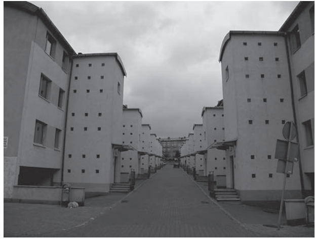
Fig. 10. Buildings at TBS at Łucznicza Street in Szczecin – condition in 2010. Photo by author
