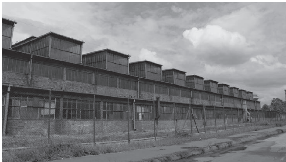
Fig. 13. Stalowa Wola, industrial halls of Metal Factory in the steel frame construction system. Photo by author, 2010
