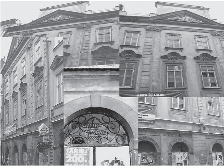
Fig. 3. House at Szczepańska Street 5, Cracow – before remodeling; former Restaurant “Pod Trzema Rybkami”
