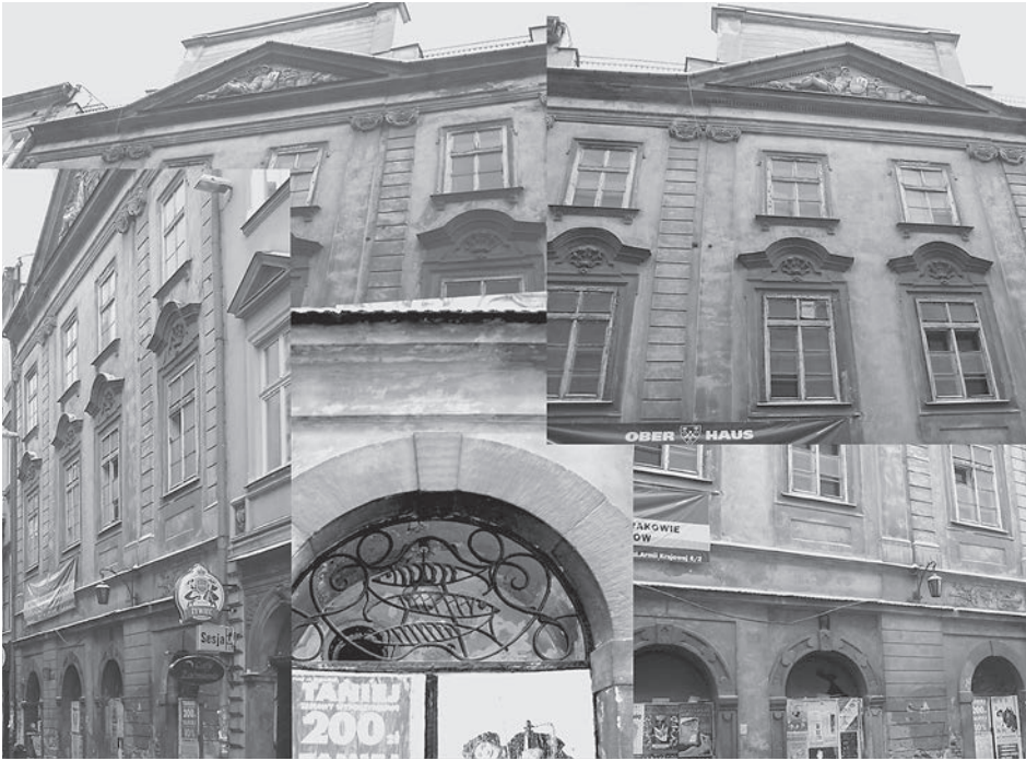
Fig. 3. House at Szczepańska Street 5, Cracow – before remodeling; former Restaurant “Pod Trzema Rybkami”
