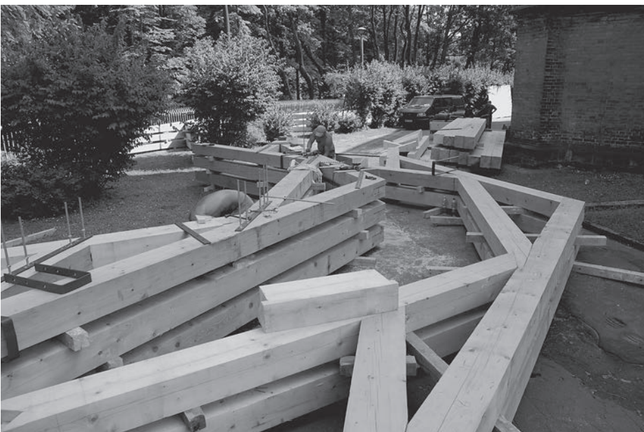
Fig. 2. Execution of the reconstructed roof framing trusses
