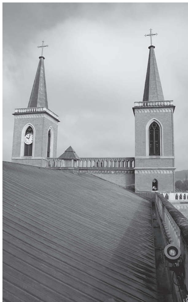
Fig. 6. Final view of the roof slope after renovation
