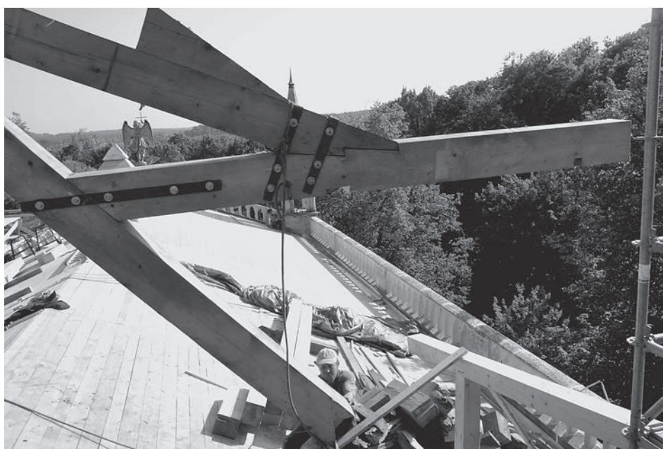
Fig. 3. Fixing the roof truss on the wall crown
